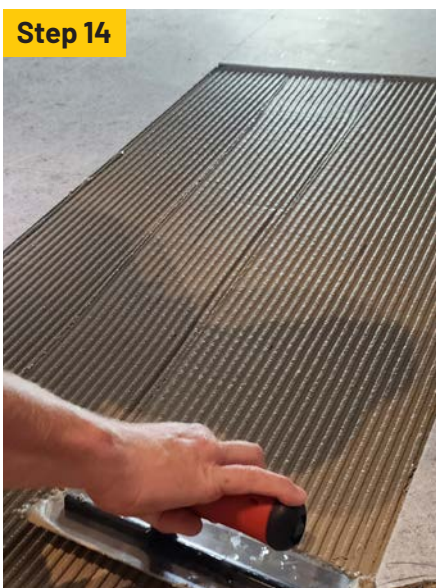
Spread the mortar one directional keeping the ridges high.
