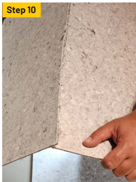
Snap and cut it from the back site.
