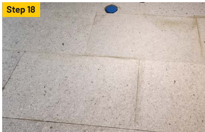
Final example of finished installation. For sound deadening installation cover all joints with 3/4" masking tape prior to tile installation.
