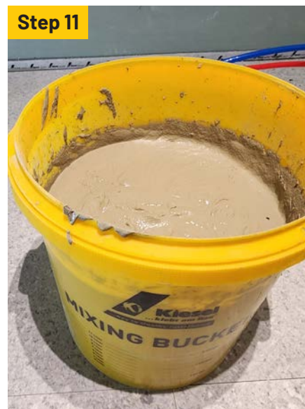
Mix Servoflex 5, Servoflex Trio SuperTec or Servoflex Pro with proper water ratio.
