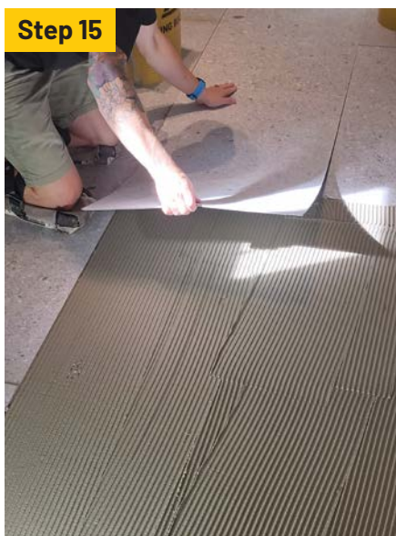
Embed OkaQuiet into fresh mortar cleaning billowed mortar between the boards.
