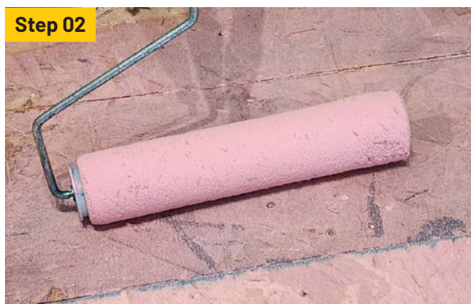
Spread Okatmos DSG over concrete or wooden substrates...
