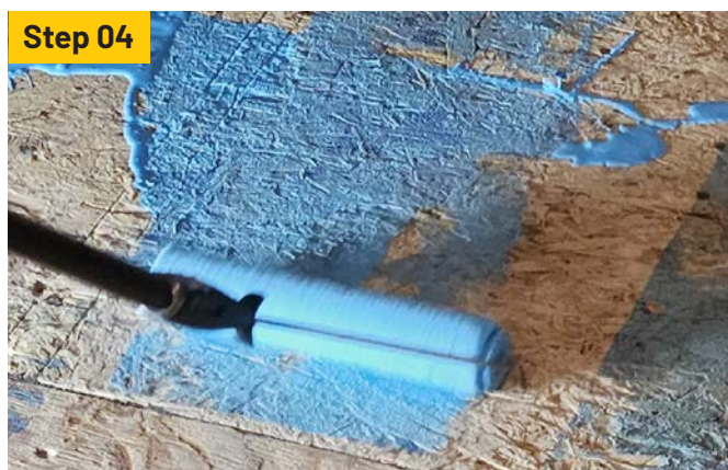
Kiesel recommends use of primers. It enhances the performance and adhesion of mortars.
