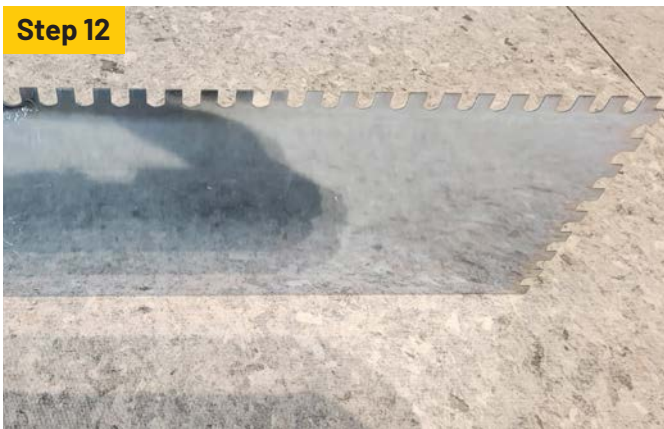
Use 1/4" x 1/4" x 1/4" square notch trowel to install OkaQuiet.
