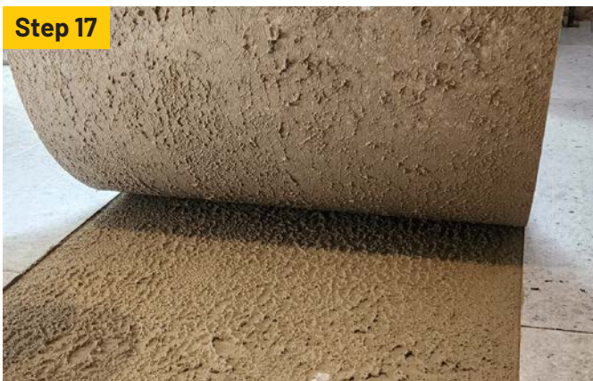
Lift OkaQuiet occasionally to check for proper coverage.
