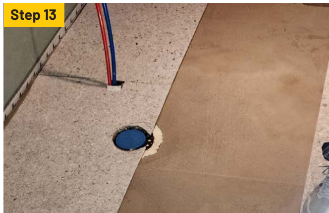
Remove loosely laid OkaQuiet within hands reach (typically one row).
