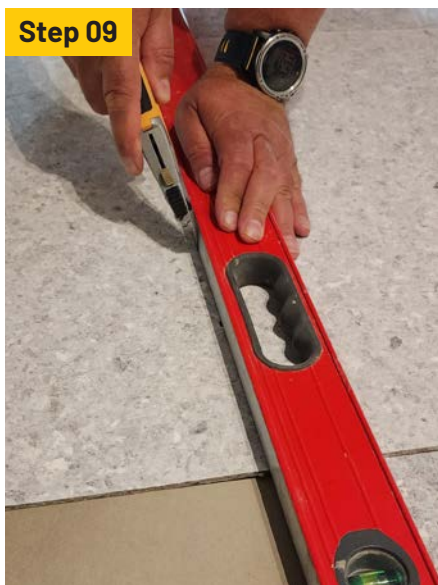
Score OkaQuiet with heavy duty utility knife.
